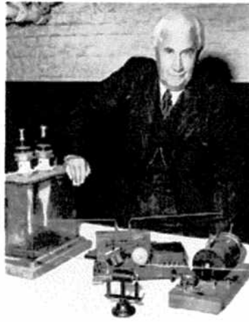
Christian Hülsmeier and his telemobiloskop. The spark gap transmitter is on the left; receiver, dipole antennas and bell on the right. Left photo was taken in 1904; right photo, considerably later. The telemobiloskop is now on display at the Deutsches Museum, Munich
